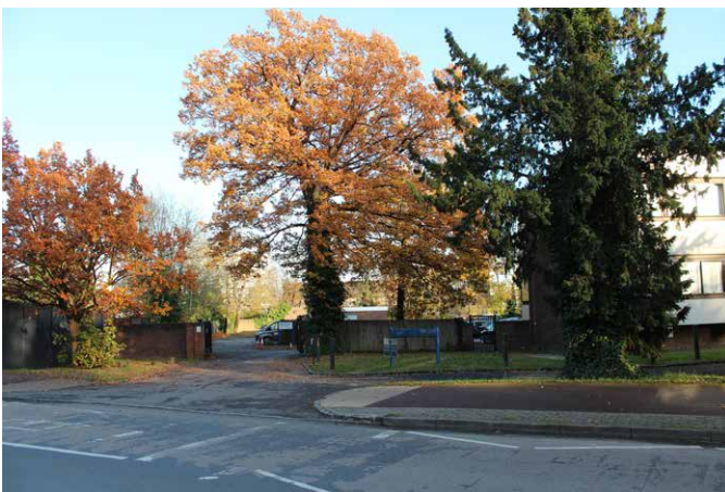
Access into Police Station (Footpath/Cycle link in front) with secure rear compound and turning for car parking to right.
